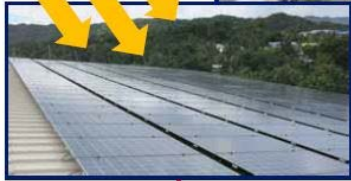
Solar photovoltaic module: Kyocera 250W x 600
