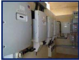
Inverter: 10kW x 15 Monitoring System
