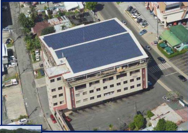
Solar photovoltaic module: Kyocera 250W x 600
