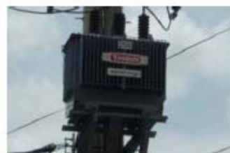
Amorphous metal transformer
