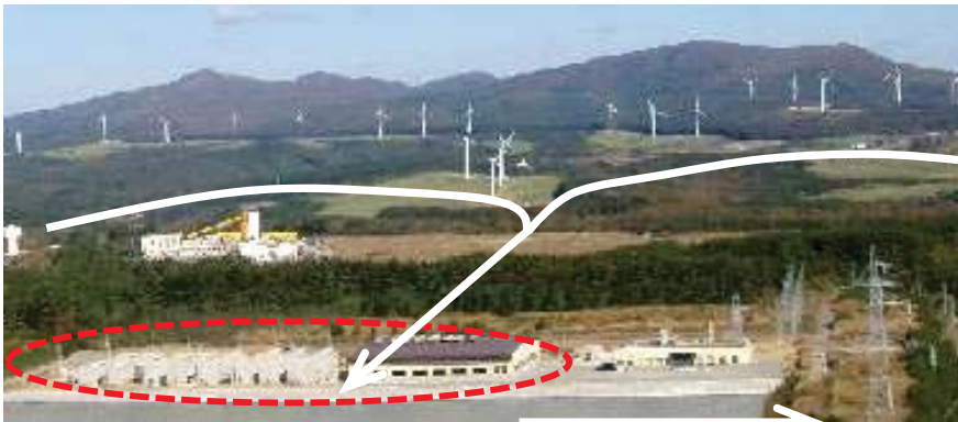
Battery Station (e.g. NAS Battery, 56MW/370MWh)
