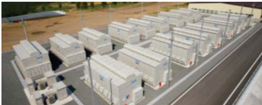
Battery Station (e.g. NAS Battery, 56MW/370MWh)
